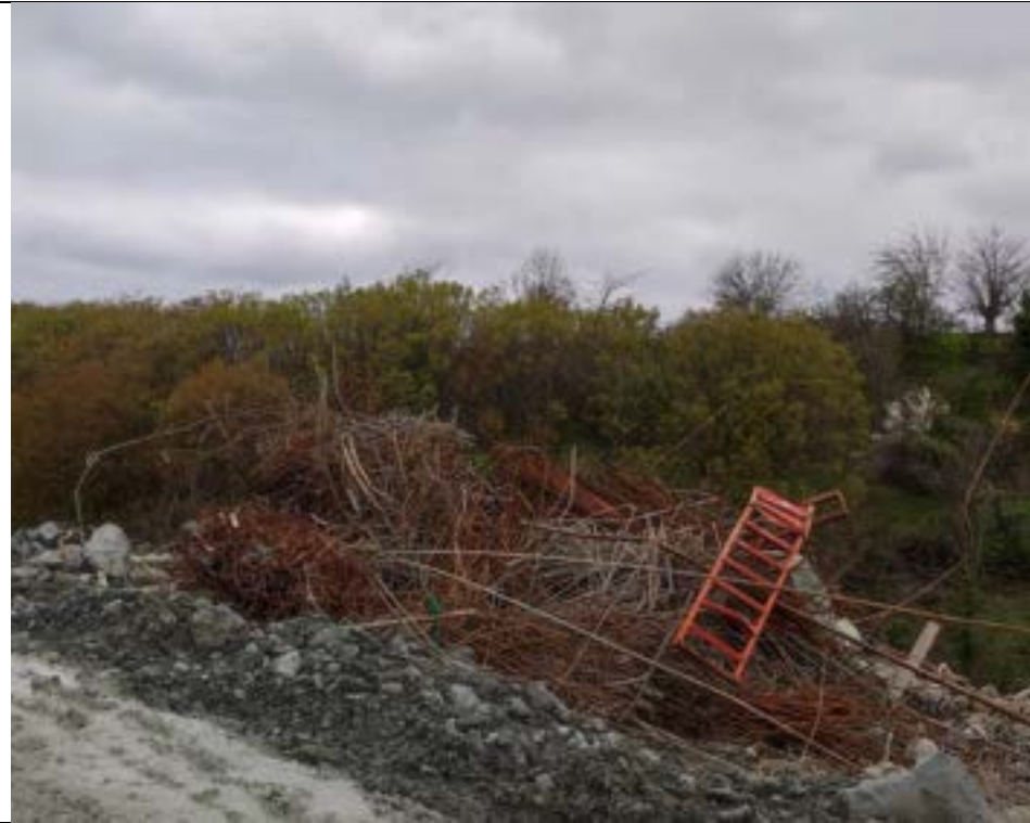
Improper Storage of Scrap Metal Waste (Tunnel 5 Argveta Site Workshop, March 2023)
