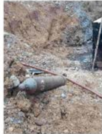
Bridge N1, pier 11
