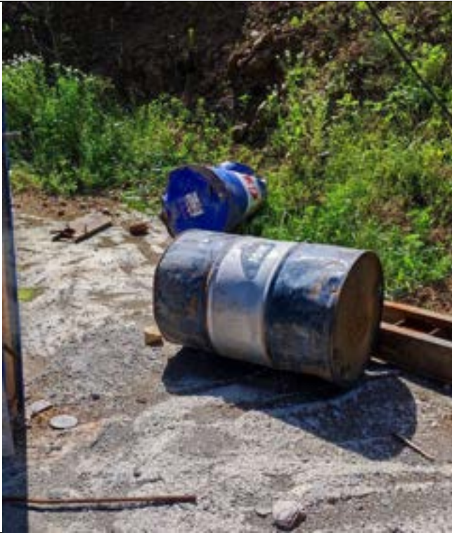
Poor Hazardous Waste Management (Tunnel 4 Portal, June 2023)
