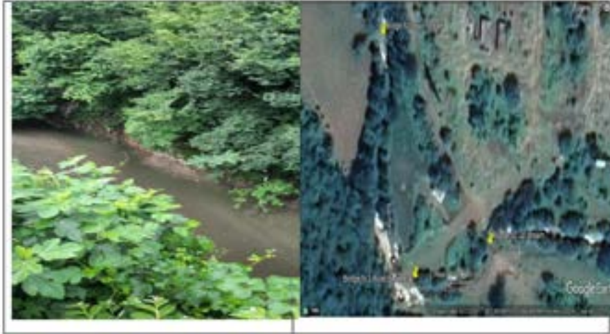
Figure 5-4 Bridge N3 downstream (Borimela River)
