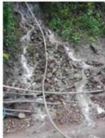
Tunnel N3 (Near the main distribution board)
