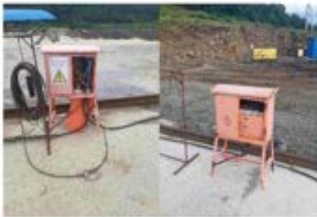
Bridge 3 (Interchange N1)
