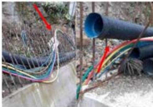
Tunnel N: 2AT-T
