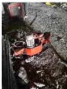
Tunnel N2AT-A – Steel cutting machine in working condition has been observed.
