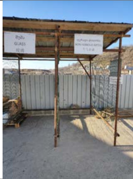
New Glass and Non-Hazardous Waste Collection Area (Next to Hazardous Waste Storage Area, January 2023)
