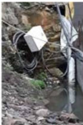
Tunnel N2 AT-T
