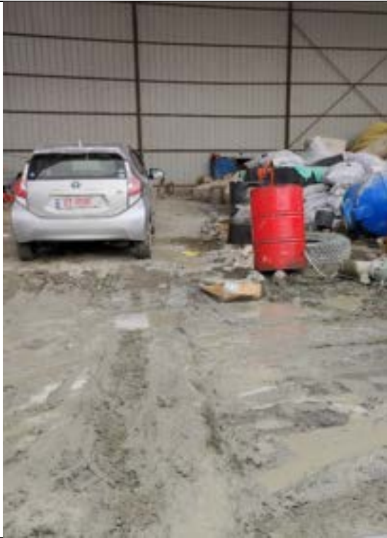
Improper Storage of Hazardous Material Container (Tunnel 5 Argveta Site Workshop, March 2023)
