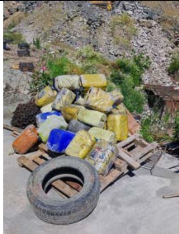
Poor Hazardous Waste Management (Tunnel 4 Portal, June 2023)
