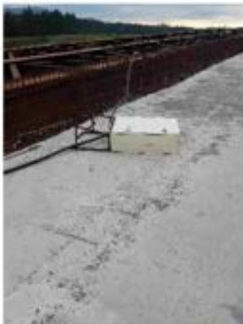
Bridge 4 (Interchange N2) – Fallen down electric box has been observed. After verbal warning, given to the Contractor's site responsible persons, it was fixed in correct position.
