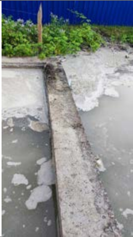
Poor Water Management in Batching Plant No 2 (June 2023)
