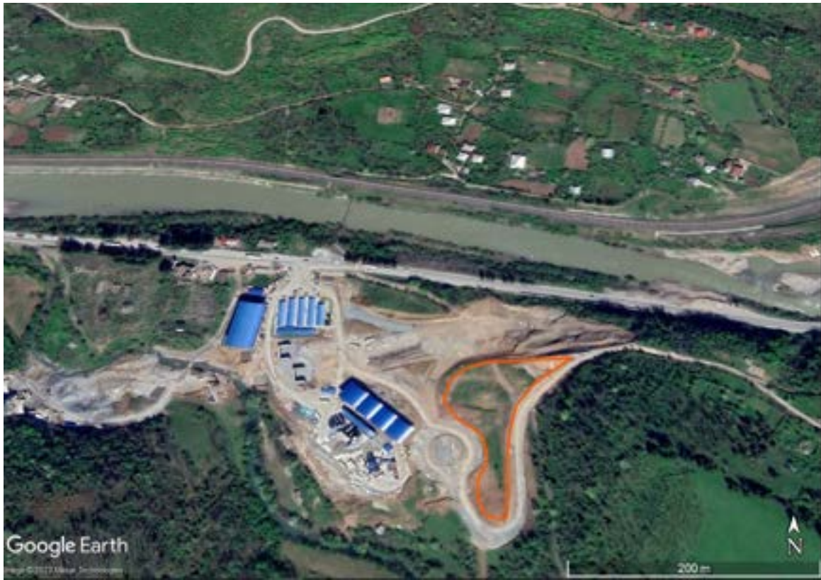
Figure 5: Proposed Planting Plot N2 near Interchange N1 (Left Bank of the River Dzirula)
