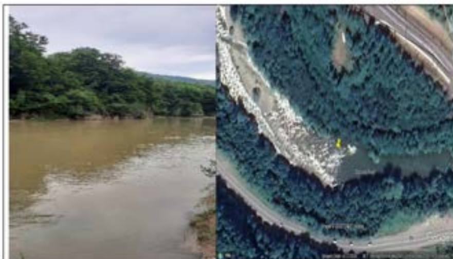
Figure 5-8 Bridge N1 downstream (Dzinula River)
