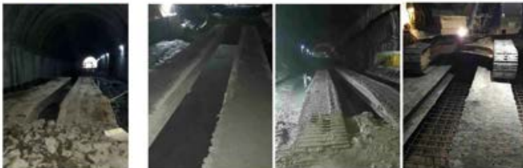
Tunnel N1 AT-A
