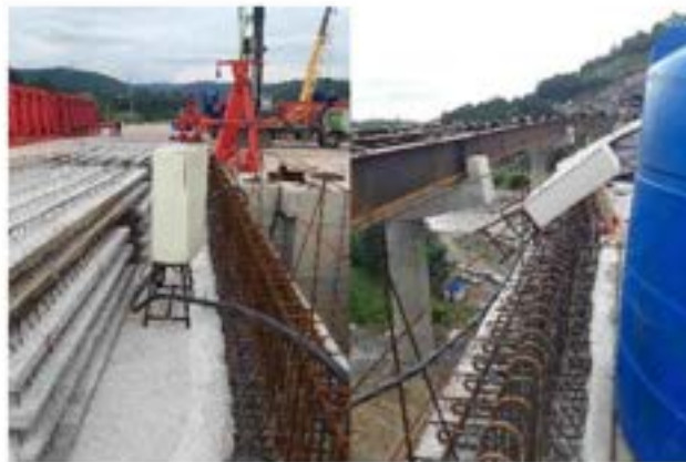
Bridge 4 (Interchange N2)
