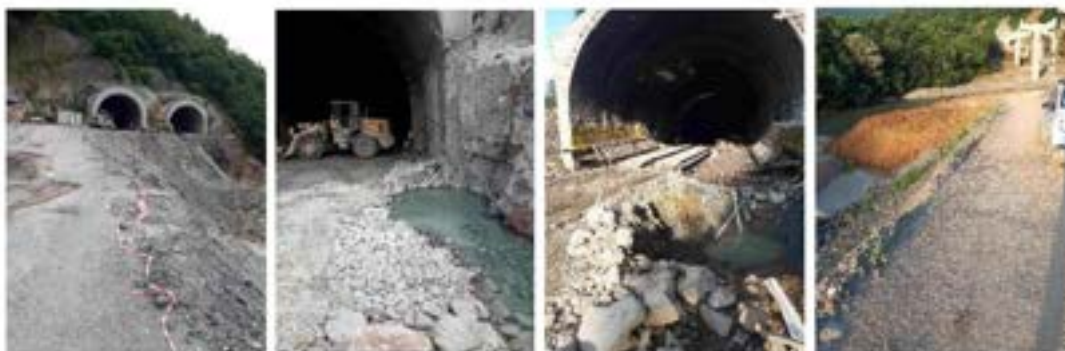
Access to Tunnel N3
