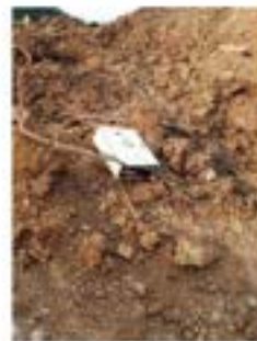
Bridge N1, pier 11
