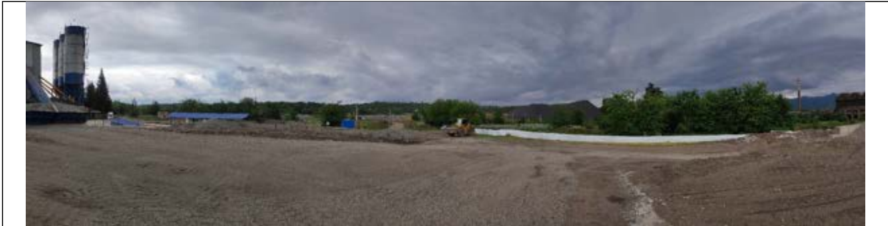
Panoramic View of Batchingplant No 2 (June 2023)
